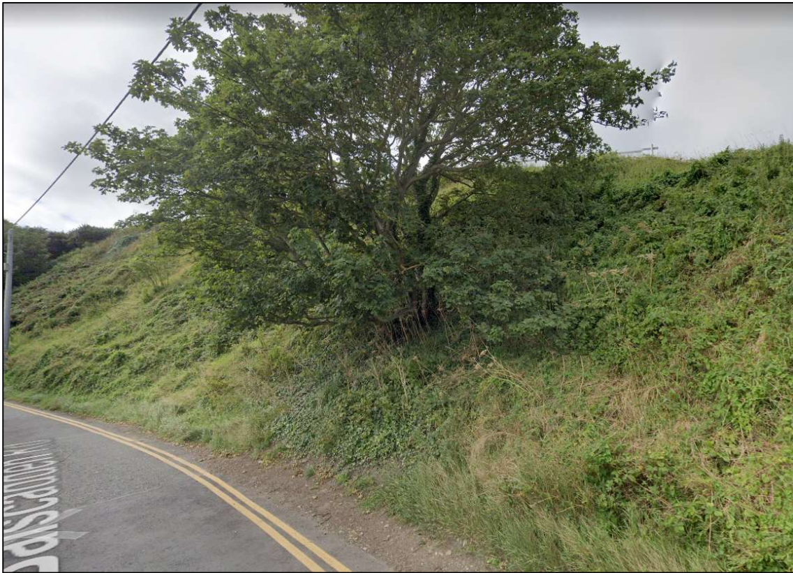
Figure 9.2: Balscadden Road adjacent to the site
